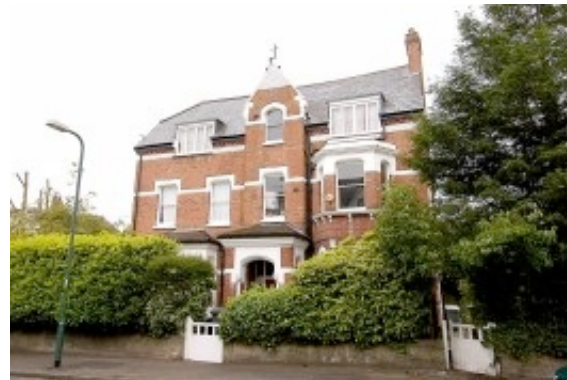
Side entrance, the gate on the right.
